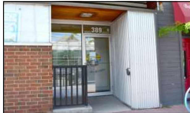
Entrance to 389 Richmond Road (Downstairs Hall)
